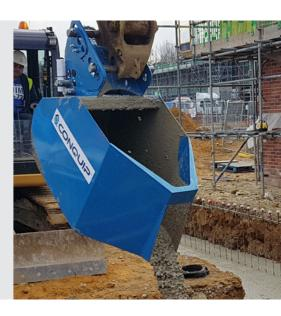
Ideal for housebuilding sites as excavators can access areas a concrete truck is unable to. Filled straight from the truck, it can pour foundations, columns, slabs and other applications.
